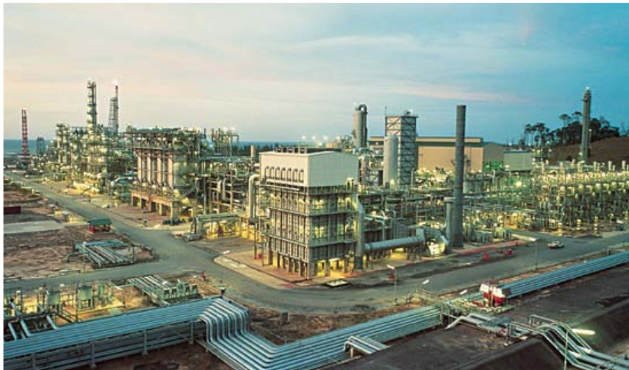
Shell Bintulu 15,000 BPD Gas to Liquids (GTL)
